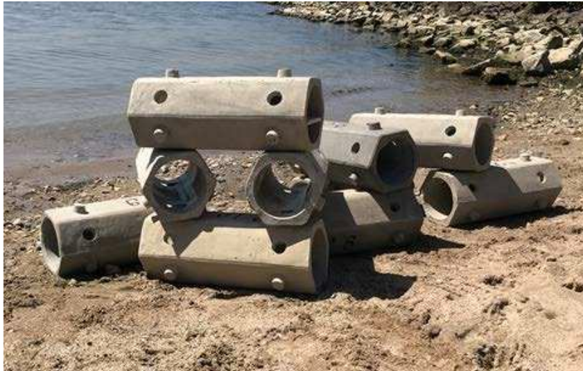
Figure 3.6. Fish hotels, an idea of Tinka Murk, Wageningen University. Structures made of concrete with large holes and interlocking system with pins aimed at large fish. (Source: Wageningen University).
